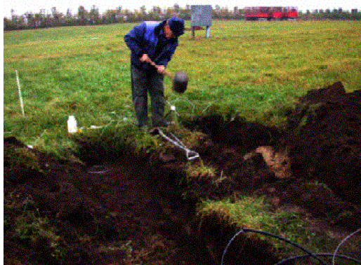
Fig. 4.1.1. Installation of Teflon suction cups in the grass-clover field.
